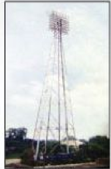
Stadium Light Tower
