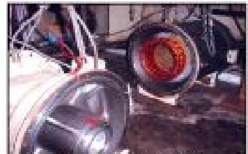
Overhauling of Central A/C system
