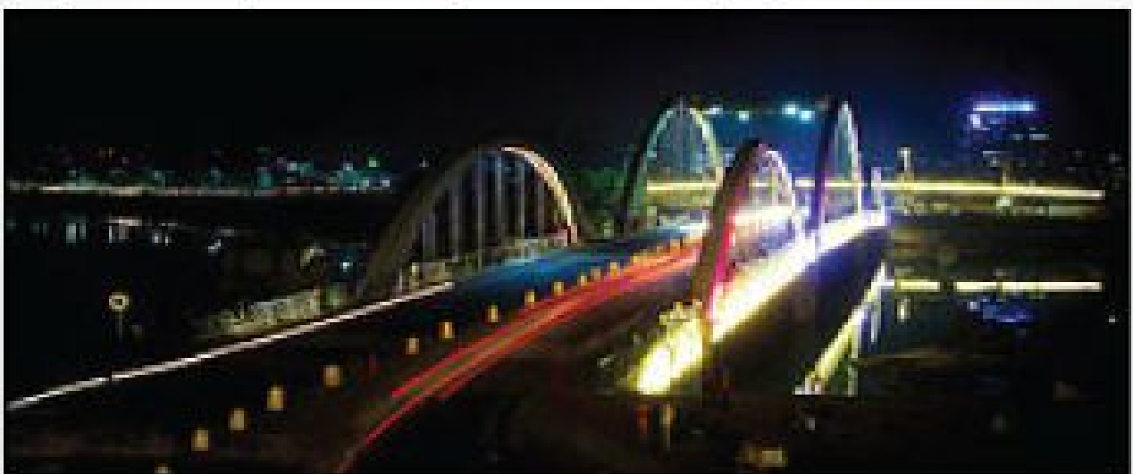
Bridge Lighting & Street Lighting Hatirjheel Area
